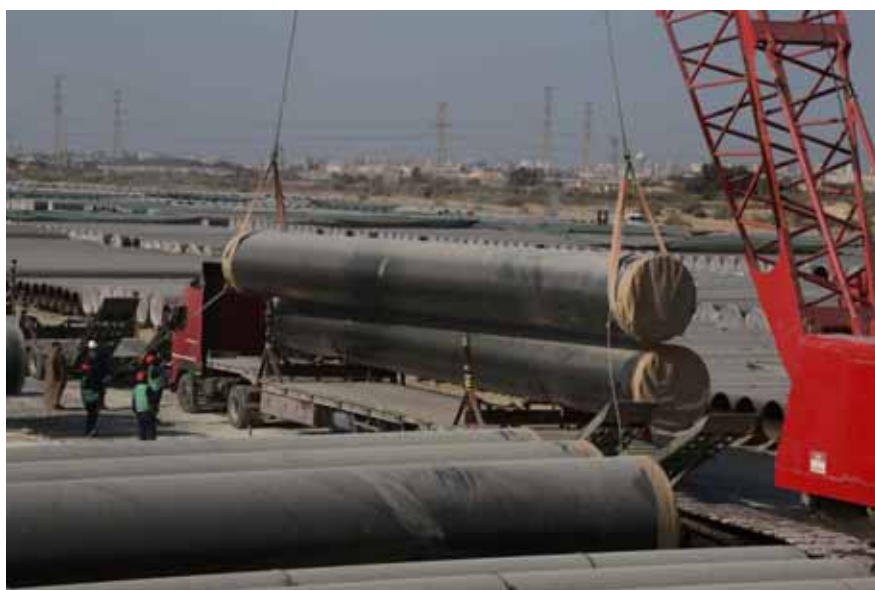
Figure 2. Pipe sections being transported.
