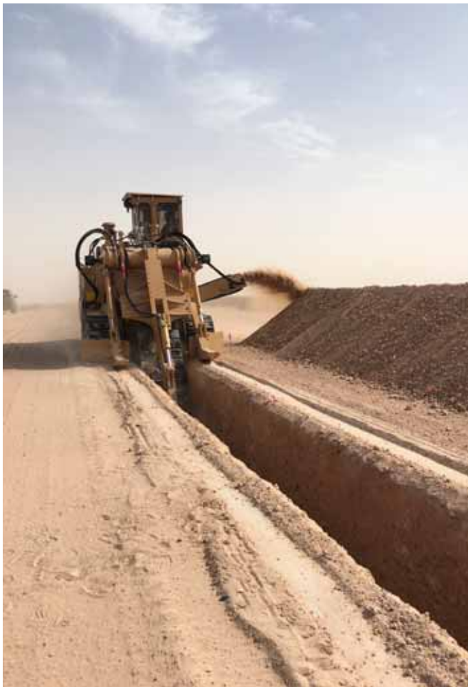
Tesmec 1150 chainsaw digging in Kuwait.
