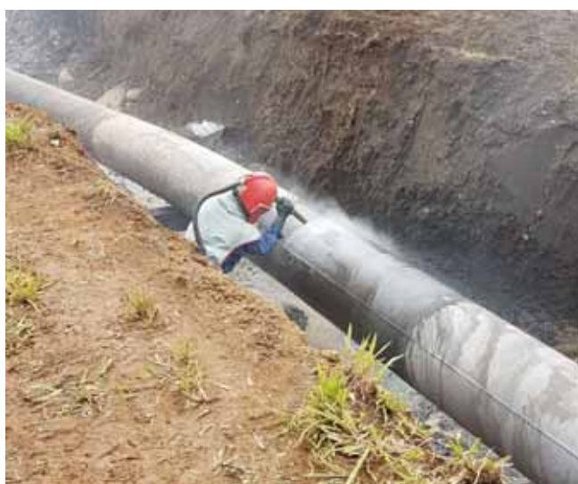
Figure 5. Vapour blasting with the approved acid salt remover.
