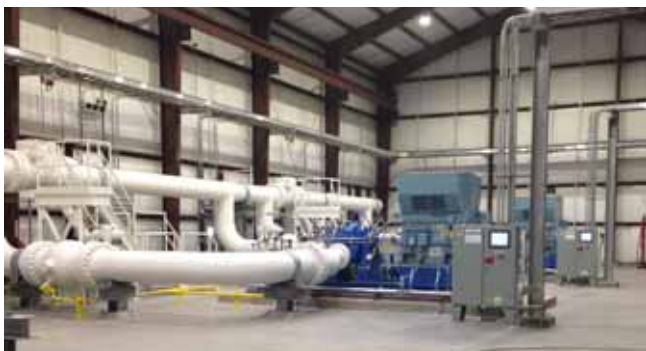
Figure 2. The project presented several challenges, including working through the winter months.
