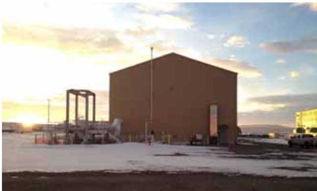
Figure 1. Detailed project planning and co-ordination ensured each aspect of the installation was completed on time.
