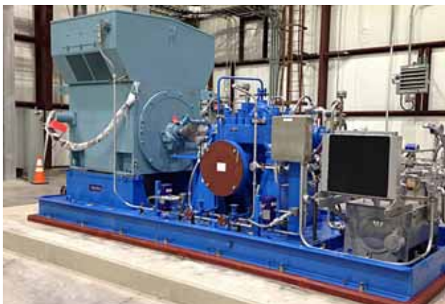
Figure 3. The completed installation will have a pumping capacity of 320 000 bpd of light crude.
