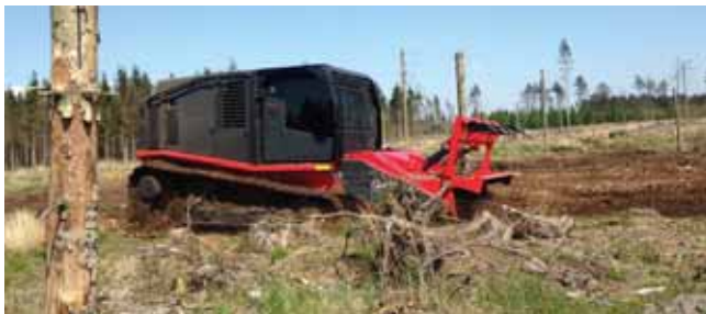
Land clearing with the RAPTOR 800.
