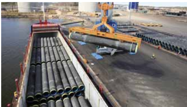
60 t Suxxesion type DEHK 600 hydraulic pipe lifter loading a supply boat with concrete lined Nord Stream pipes suspended from a Liebherr HMC 550.
