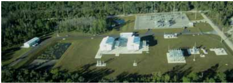
Figure 3. Aerial view electric powered compressor station.
